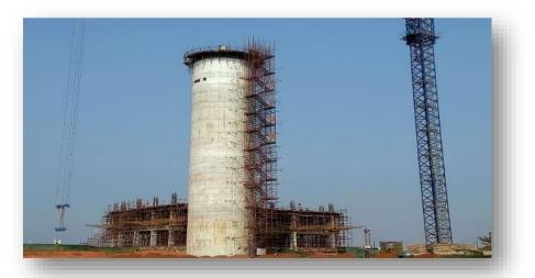
Airport will have state of the art ATC tower with modern facilities and equipments. The ATC centrally located towards west of the terminal building, is provided with a ground level entrance, tower level 1 will be technical, tower Level 2 will be technical and support (break room) and tower level 3 will be the control room. The cabin for the air traffic controllers is designed as a rounded structure to allow for almost 360 degree view of the aerodrome.
